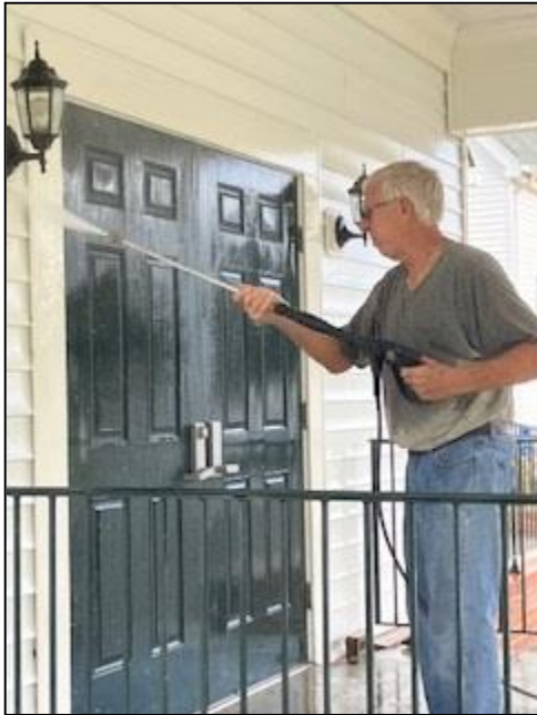
Pressure washing the doorways
